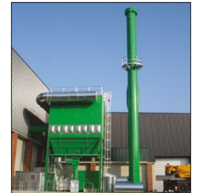
Filter unit with burst disks
